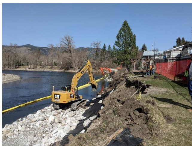
Installation of revetment on the Kettle River to curb erosion after 2018 and 2020 freshets.
