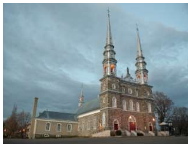
Heritage buildings at risk of flood damage in L'Islet
