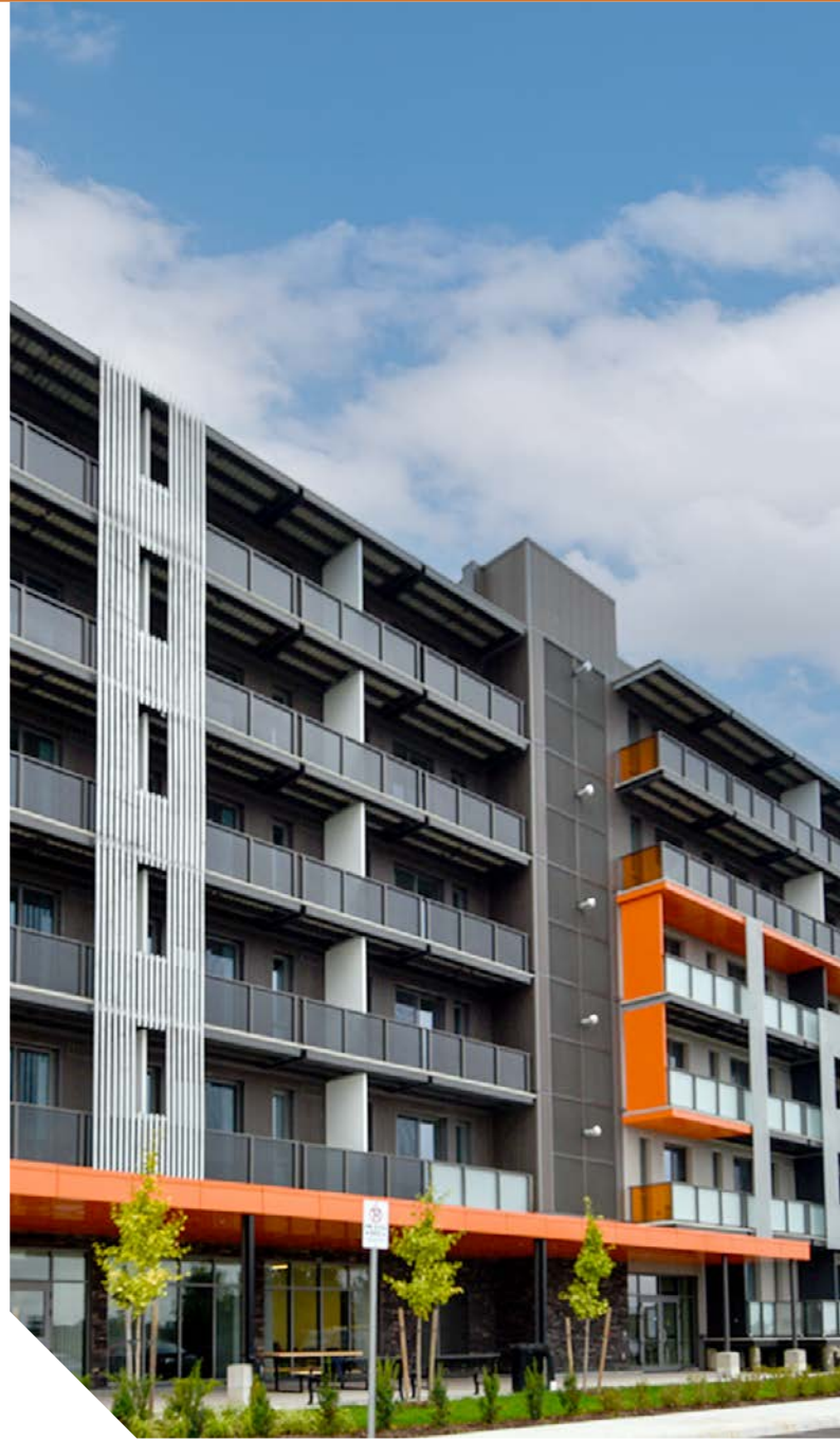
FUZE Woodstock, Woodstock, ON. A 183-module, 92,000 sq. ft. multifamily project designed by Skyhook Modular with affiliates Z Modular Holding Inc, Melloul Blamey Construction, Entuitive and Quasar.
