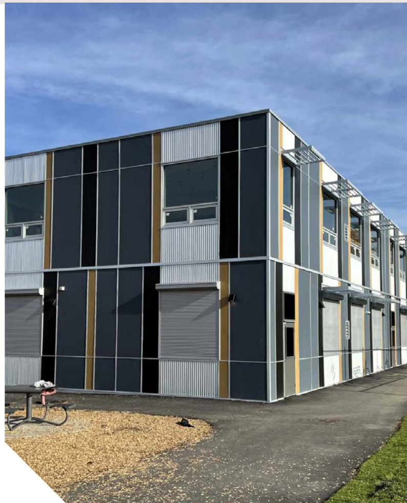
Lynn Fripps Two-Storey Permanent Modular Addition, Langley Twp, BC. An 18-module, 9,900 sq. ft. educational facility built by Fort Modular Inc.
