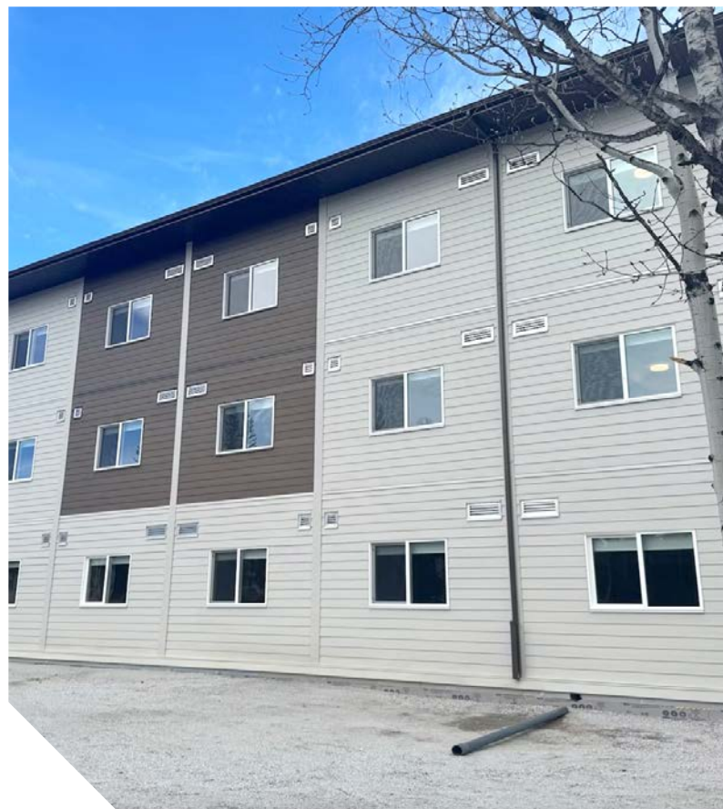
Pomeroy Lodging Employee Housing, Kananaskis, AB. A 36-module employee housing complex built by ROC Modular with affiliate Steenhof Building Services.
