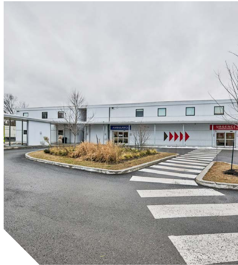
Hôpital Générale du Lakeshore Modular Complex (Lakeshore General Hospital), Pointe-Claire, QC. A 48-module, 32,000 sq. ft. addition to an existing hospital built by ATCO Structures & Logistics Ltd. with affiliate CIUSSS de L'Ouest-De-L'Île-De-Montréal.
