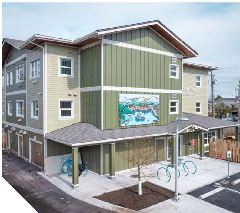
Steveston Highway Affordable Housing, Richmond, BC. A 33-module, 20,750 sq. ft. permanent affordable housing complex built by ROC Modular with affiliate Buttcon Limited.
