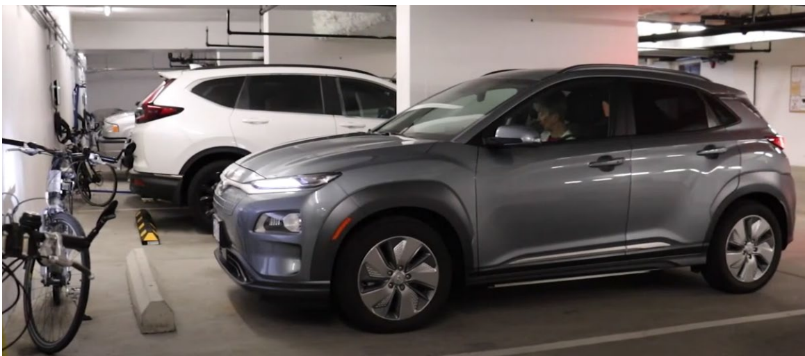
Figure 1. EV Charging in a condo building in Saanich, BC (on the left wall). Source: District of Saanich
